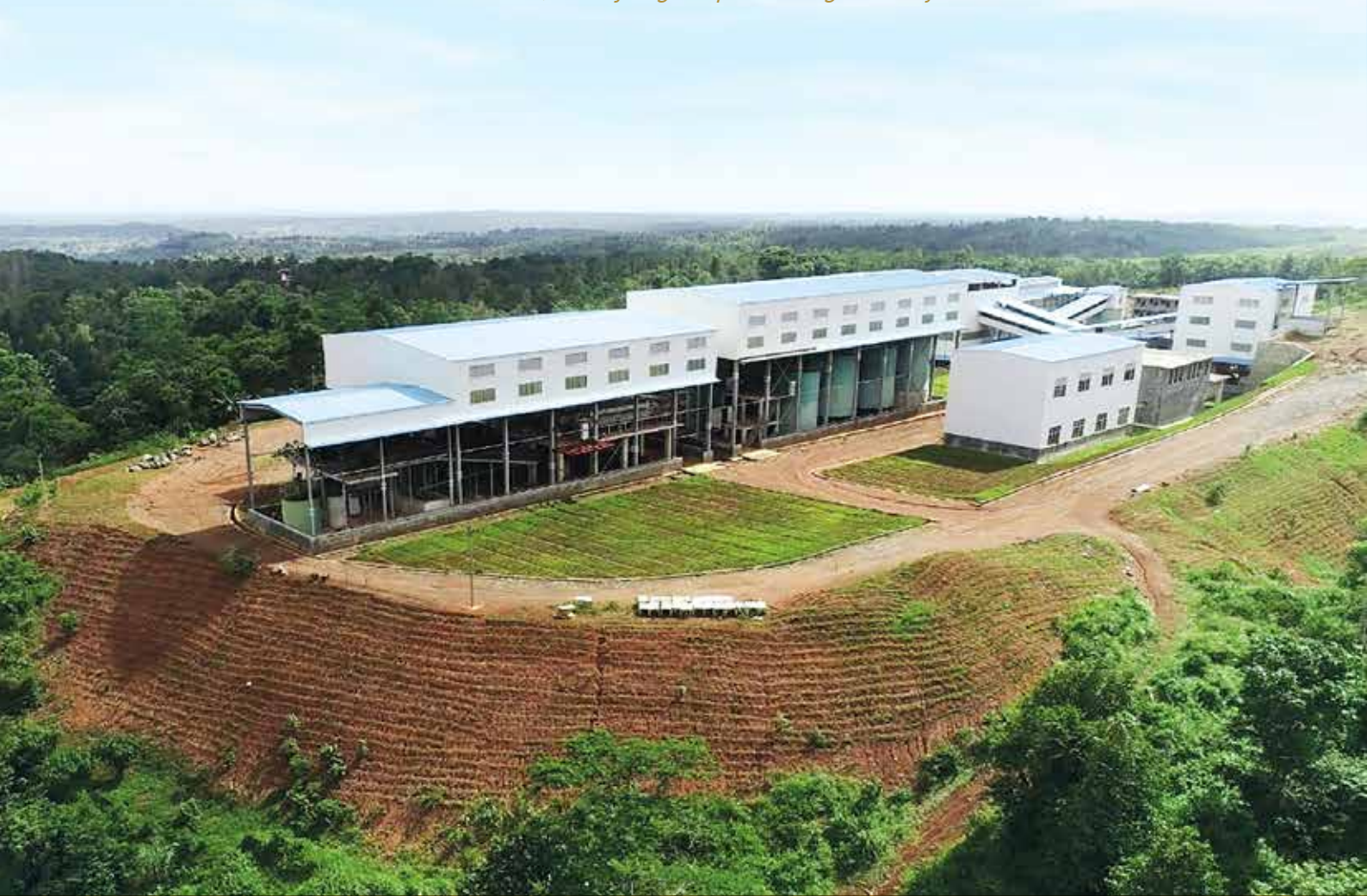
Tampilan keseluruhan dari fasilitas pengolahan floatation and carbon-in-leach berkapasitas 500 ton per hari Overall view of the 500 tonnes per day floatation and carbon-in-leach processing facility
